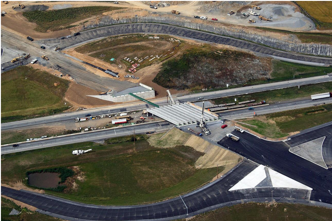
An aerial image of the SR1002/33 Chrin Interchange Project during construction.
