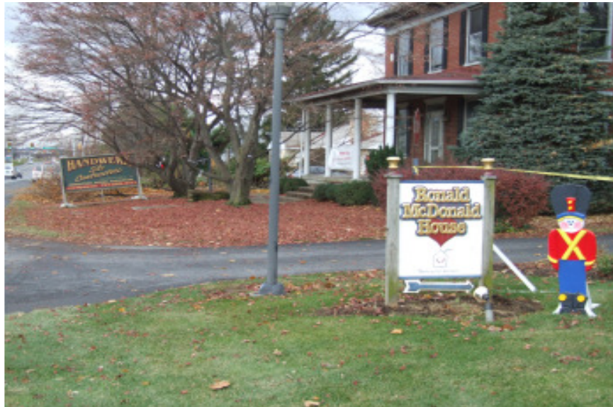
The existing structure (behind The RMHC sign) before the demolition which will allow for expansion of the current RMHC facility.
