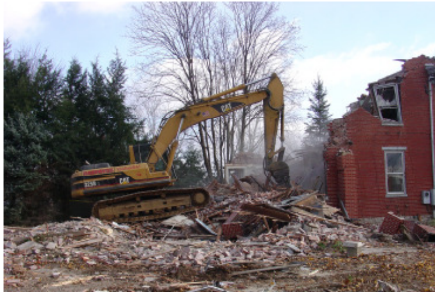
A Handwerk Trackhoe dismantles existing structure on proposed expansion property.
