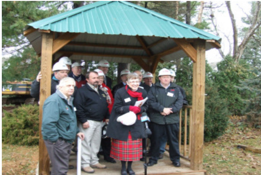
Representatives from Gilbane Building Company, Handwerk Site Contractors, and Frescatore Consulting, Inc., with Kathy Denton of RMHC (front), on the demolition site.
