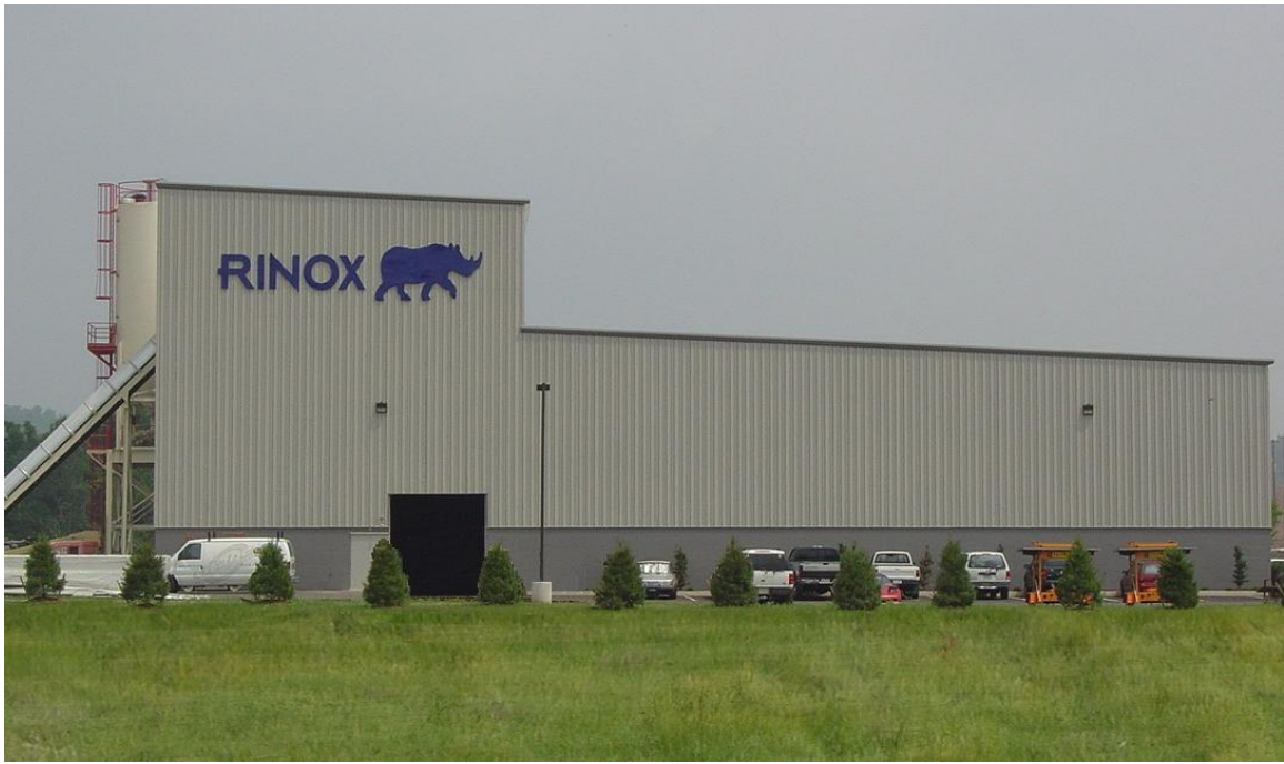
Photograph of RINOX' s 35,000 square foot manufacturing facility as seen from Benjamin Franklin Highway in Douglassville, PA.
